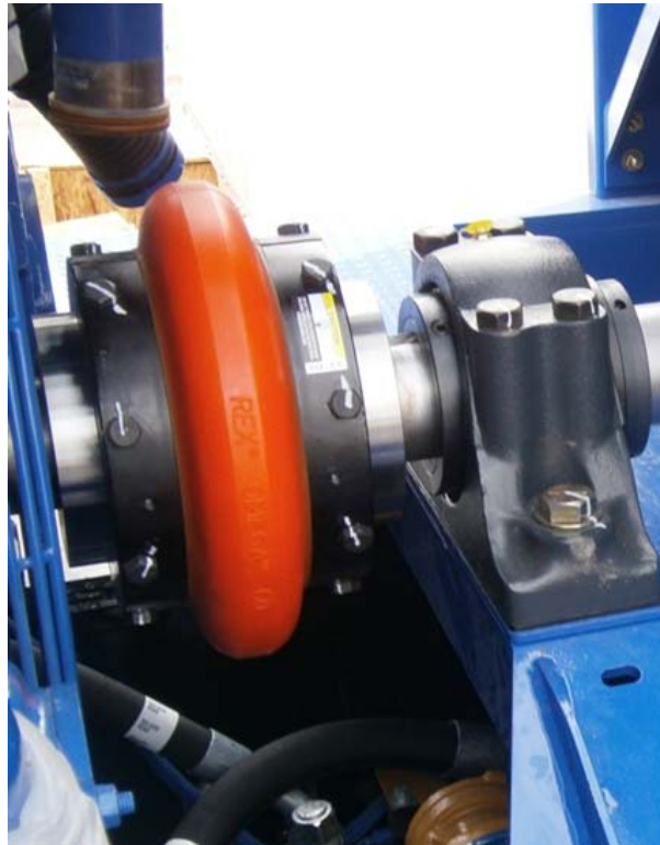
Figure 14: Flexible coupling installed
